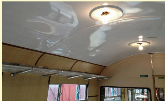
Completion of replacement ceilings and Formica panelling in W51073, along with refitted original components such as luggage racks and alloy trim.
