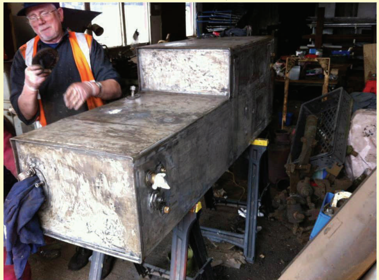
51503's fuel tank number 2 being stripped ready to have its leak repaired
