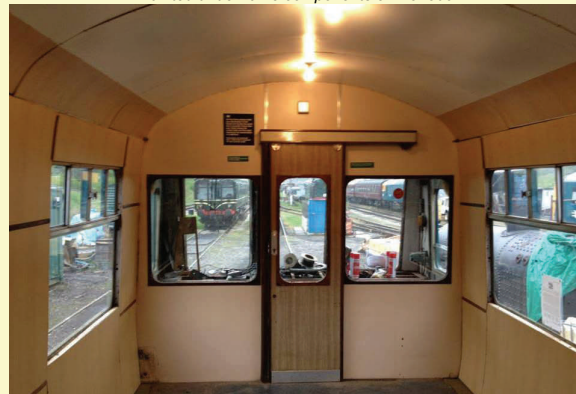
New panelling installed into the "First Class Smoking" saloon (at the front of the vehicle) in W51073. Original Formica can be seen in the form of the refurbished sliding door, now also refitted.
